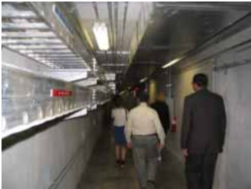
Access tunnel at the Pocahontas Parkway facility
