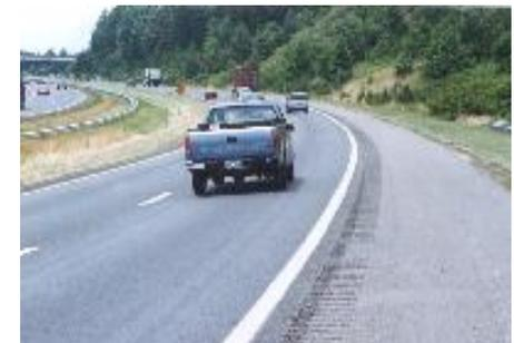
*Paving shoulders, improving clear zones, better retroreflectivity striping and edge-line rumble strips are all effective lane departure crash countermeasures*
